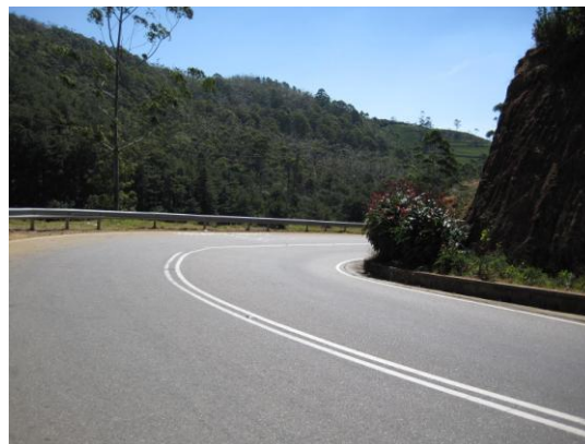
Photo 2: Improved Road Alignment (Route AA005)
