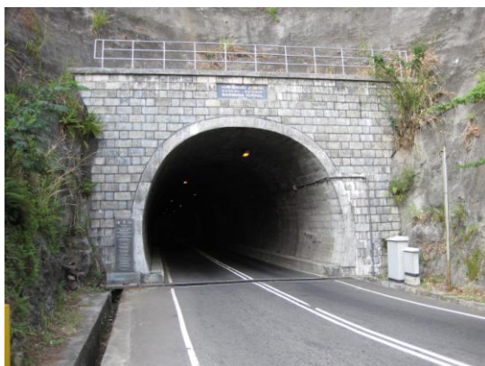
Photo 1: The Only Tunnel on National Highways in the Country (Constructed in This Project)
