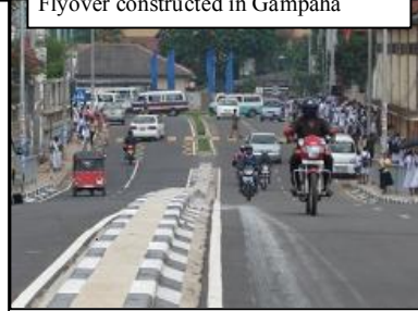
Flyover constructed in Gampaha
