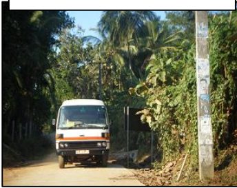
Bus operating on the improved road
