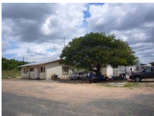
MR5 Road Depot near Sihoye
