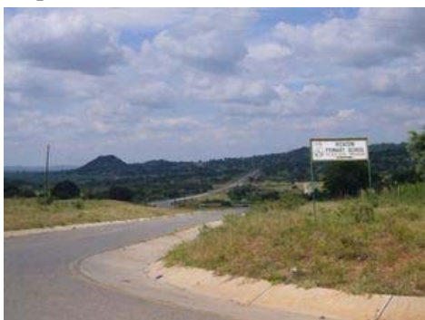
MR6 Access road (additional work)
