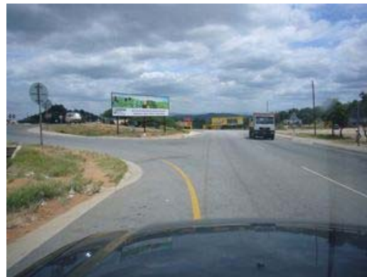
MR5/MR6 branching point (Madlangampisi) After the project
