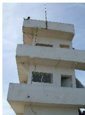
Observation tower rehabilitated by the Project (Béja)
