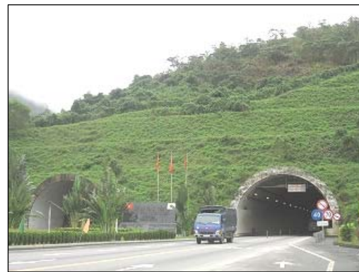
Main Tunnel (right) and Evacuation Tunnel
