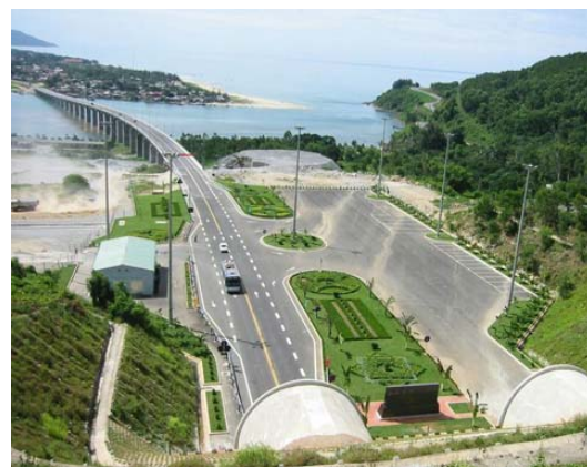
North Tunnel Section and Lang Co Bridge (Photograph provided by PMU85)
