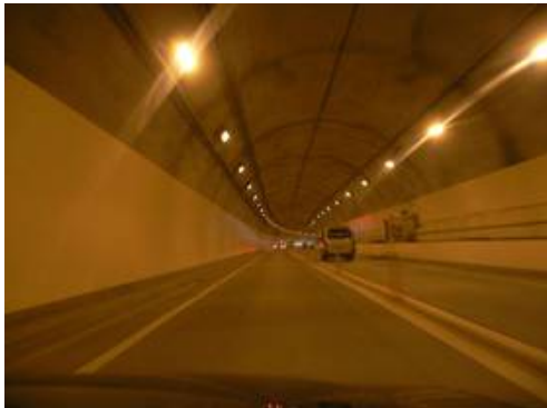
Conditions inside the tunnel
