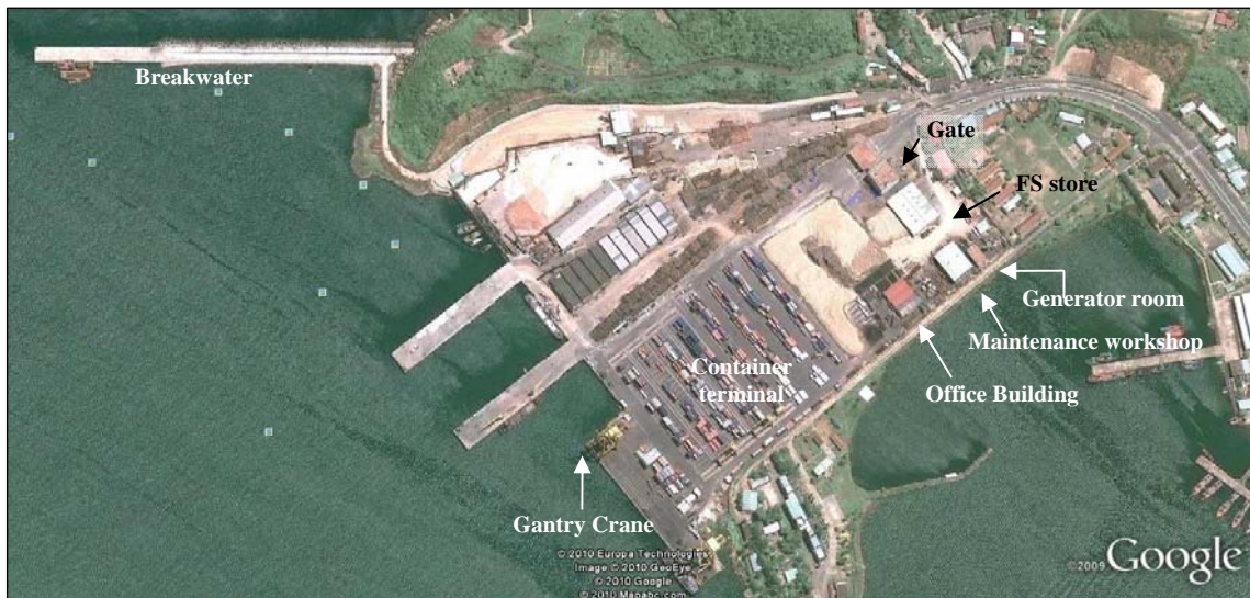
Figure 3: Key construction at Tien Sa Port
