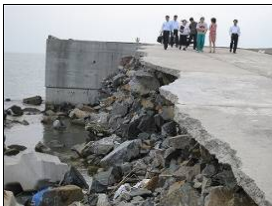
Damaged Breakwater
