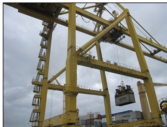
Operation of the gantry crane
