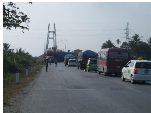
An overloaded truck, which failed to move up the approach to Kien Bridge, was stranded
