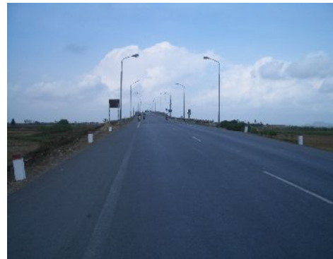
National Highway No.10
