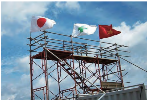
Wind whipped ‘Flag of the Safety’ in Package 1 site
