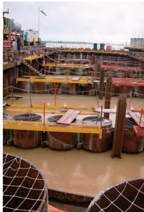
Net for falling prevention and unit scaffold
