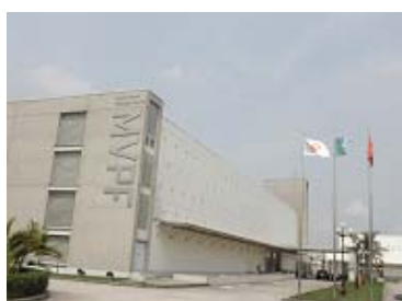
Front of the MVPF Building
