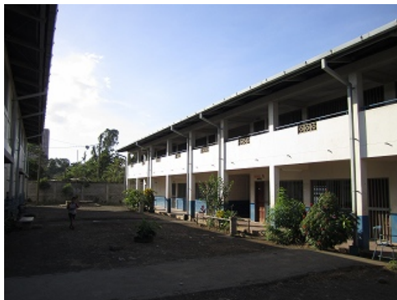
Two-story school building constructed by the Project (Alemania School, Managua City)
