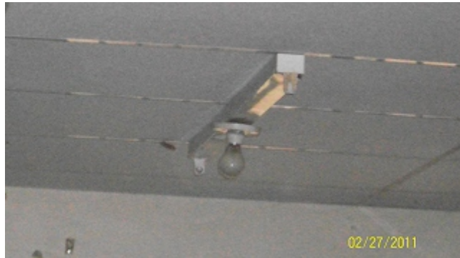
The fluorescent was gone and it is replaced by a bulb because it is cheaper (Diriangén School). This is observed at other many schools.
