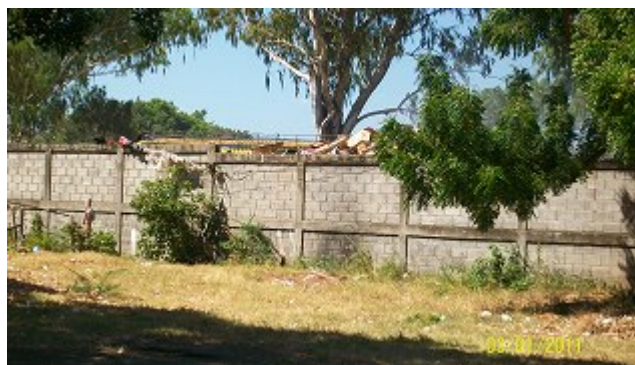
Many schools want to have high walls for security reasons as this (Fernando Gordillo Cervantes School in Managua City).
