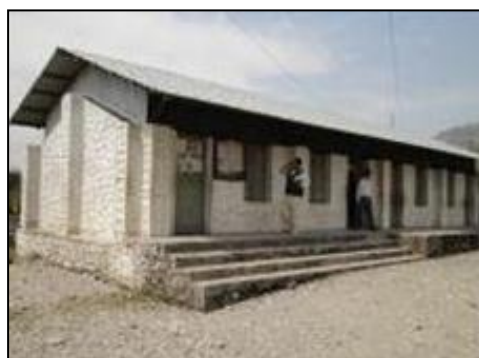
Classroom Constructed in the Project (Makawanpur District)
