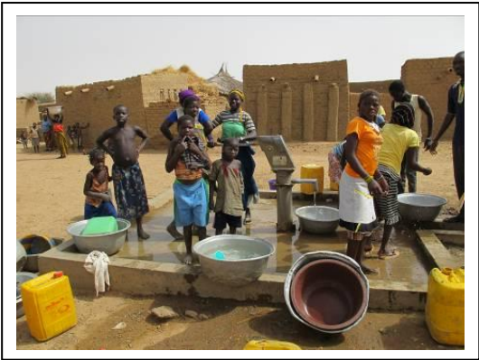
The project borehole with a hand pump
