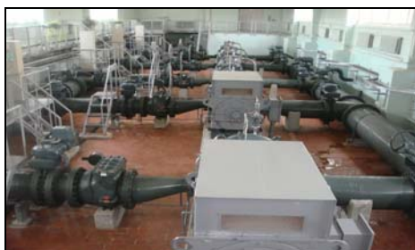
Transmission pump at upper source
