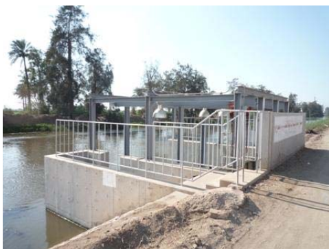
Water Intake Facility
