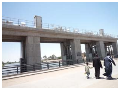
Gates and Attached Bridge
