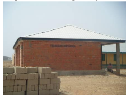
Photo: Classroom constructed by a SUBEB (Kaduna) by adopting JICA's design
