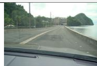
Malakal Causeway (After the renovation of pipe explosion)
