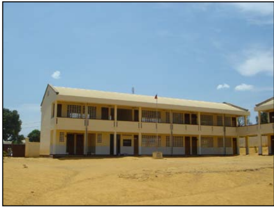
External appearance of a constructed school building (Primary School of Ebolowa in South region)
