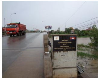
Prek Ho Bridge
