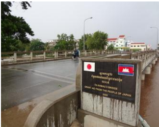
Ta Khmau II Bridge
