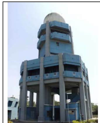
Khepupara Radar Station
