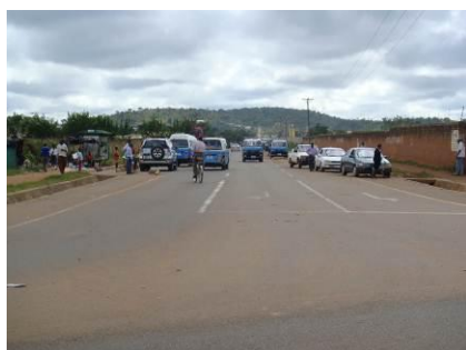
Bauleni Road. This road leads to community market and schools. Road is effectively used as Public Bus route (Blue mini-buses are shown). The project roads are generally well maintained.
