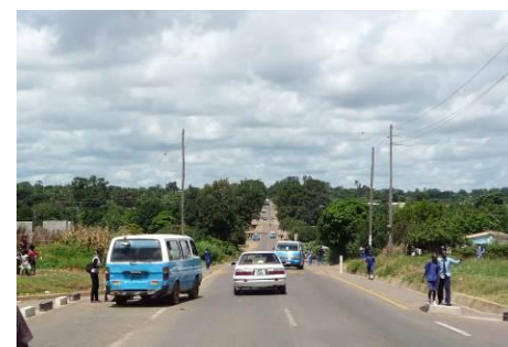
Chitanda Road. This road leads to schools. Road is effectively used as Public Bus route (Blue mini-buses are shown) and providing safety to the students. The project roads are generally well maintained.
