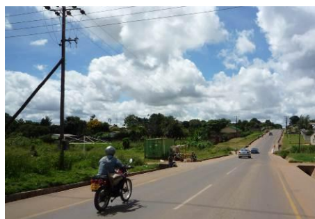
Kasangula Road. This road is effectively functioning as by-pass between two trunk roads within the Lusaka City. The project roads are generally well maintained.
