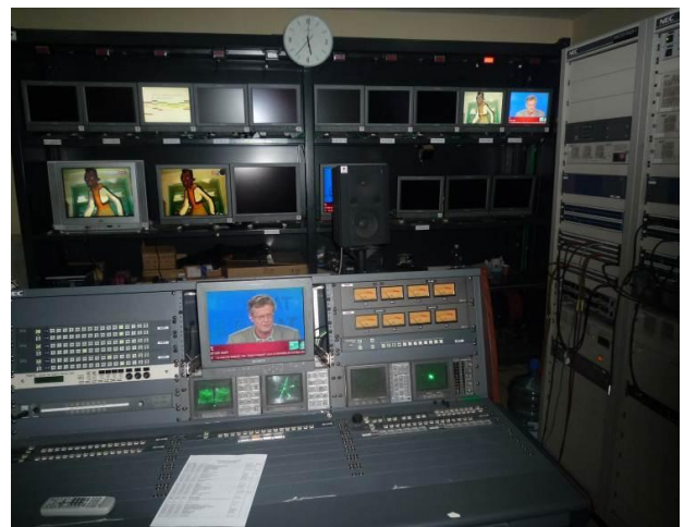
Main Control System replaced by the Project
