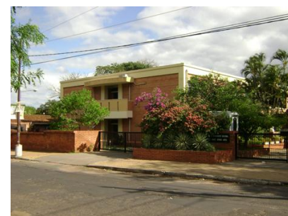
Printing and Computer Building
