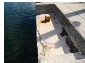
Partially delaminated concrete
