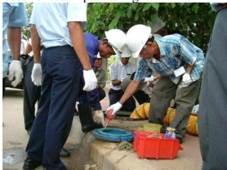
OJT on the maintenance of distribution facilities
