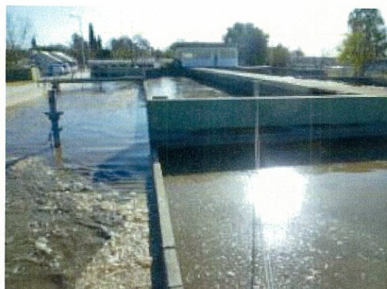
Photo 3 Hurlingham Disposal Plant
