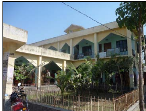
Photo 2: Union Parishad Complex
