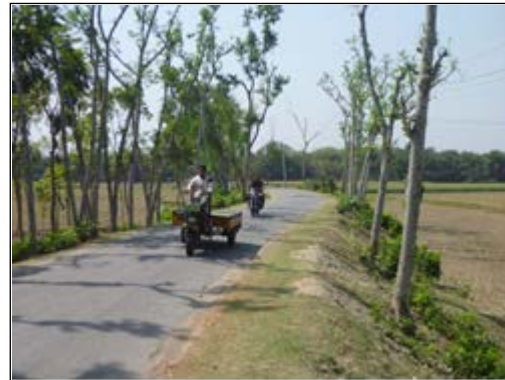
Improved Upazila Road (Rajibari District)
