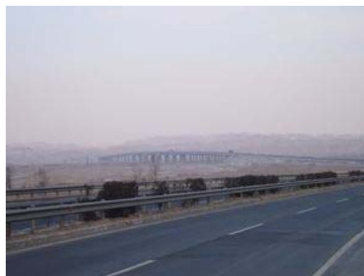
Liuzhaike-Baiyin Expressway Crossing over Yellow River
