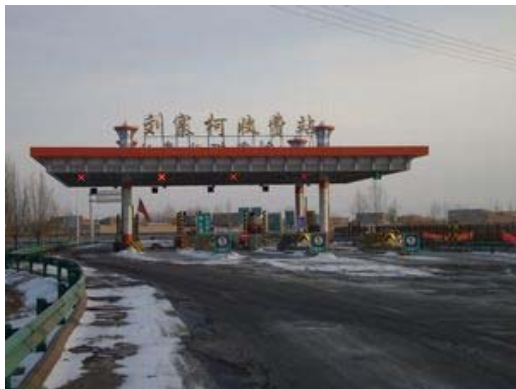
Liuzhaike-Baiyin Expressway Liuzhaike Toll Station
