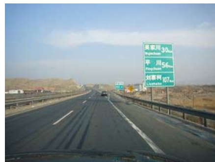
Liuzhaike-Baiyin Expressway at Baiyin
