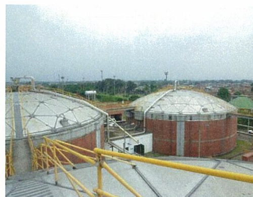
Overview of the sewage treatment plant
