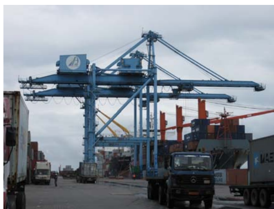
Gantry Cranes in Operation
