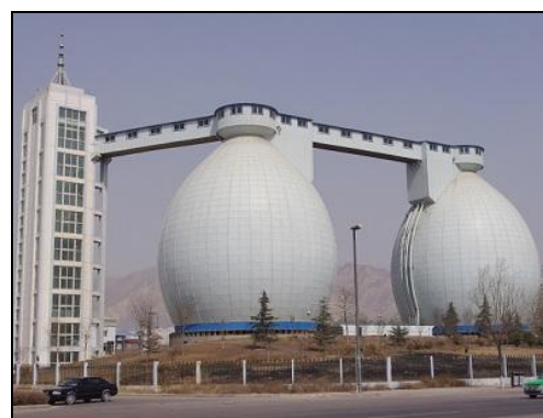
Fig. 13 Sludge Processing Facilities
