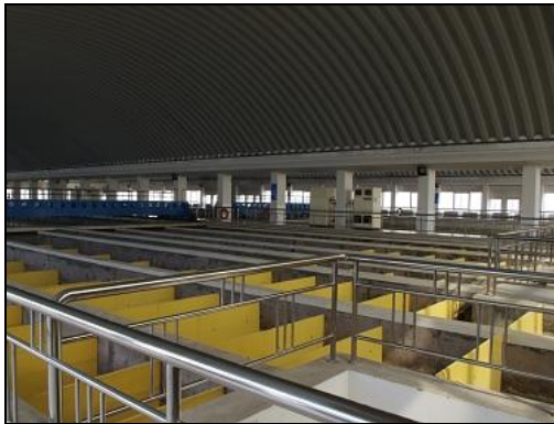
Fig.4 Water Supply Expansion Project Inside the Water Treatment Plant
