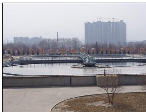
Sewage treatment plant (final settling tank)
