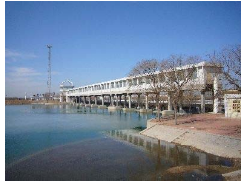
Underground Dam in Laizhou (New Construction)
