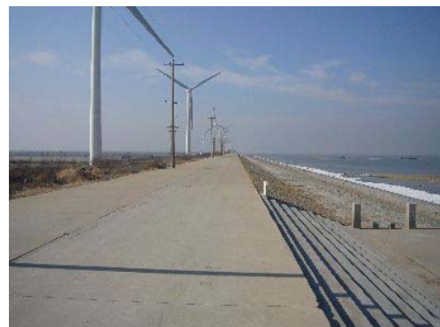
Coastal Levee in Laizhou (Rehabilitation Work)
