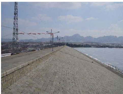
Wangwu Dam in Longkou (Rehabilitation Work)
