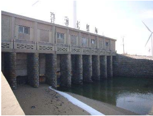
Water Gate in Laizhou (New Construction)
