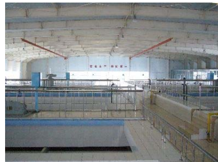
Yantai Economic & Technology Development Zone: No.2 Purification Plant
