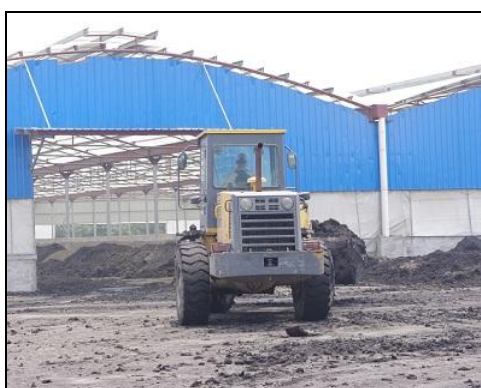
Fig. 13 Sludge Treatment in Changshu
