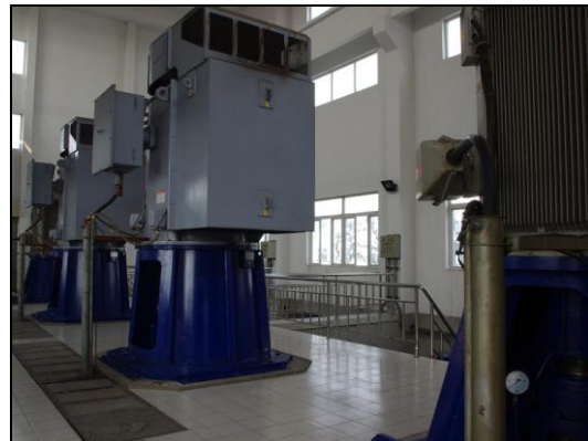
Fig.7 Intake Pumping Station
