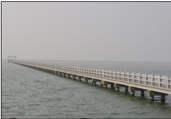
Fig.6 Water Intake at Lake Tai Shore
