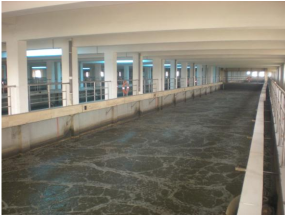
Fig. 2 Aeration tank(Hangzhou Sewage Treatment Plant)
