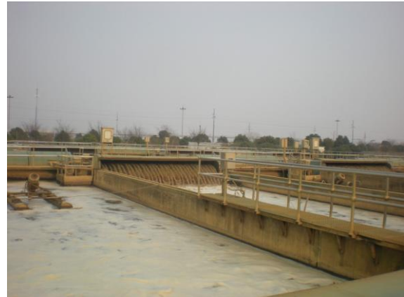
Fig. 3 Oxidation ditch (Jiaxing Sewage Treatment Plant)
