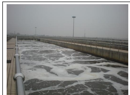
Shaoxing Sewage Treatment Plant
