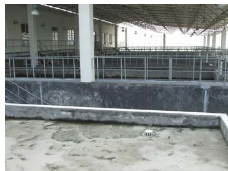
Water purification plant (Plant C)
