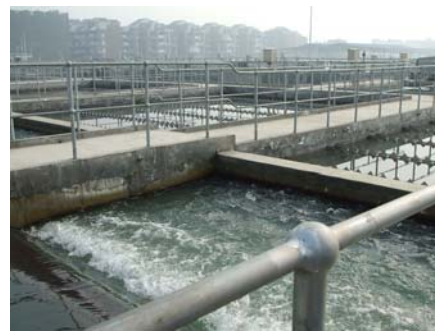
Plant C, Chengdu Sixth Water Purification Plant
