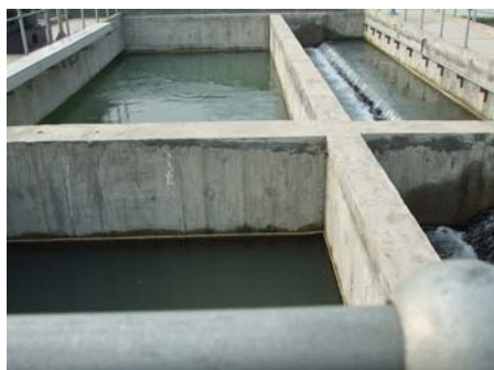
Water purification plant (Plant C)
