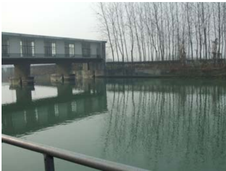
Water intake point
