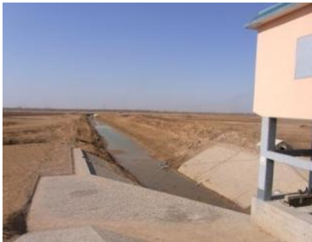
Fig.4 Main irrigation canal and pump facility in the Xiazhen area
