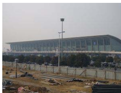
Xian Xianyang Airport No. 2 Terminal
