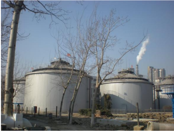
Fig. 13 Sludge digester chamber 35 (Jizhuangzi Sewage Treatment Plant)
