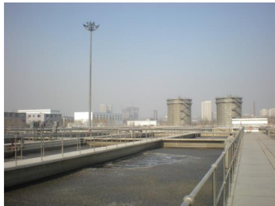
Fig. 3 Xianyanglu Sewage Treatment Plant aeration tank
