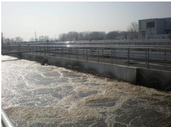
Fig. 2 Jizhuangzi Sewage Treatment Plant aeration tank
