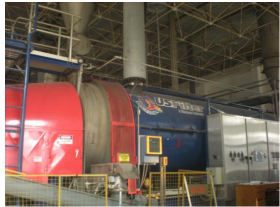
Fig. 14 Sludge dryer (Xianyanglu Sewage Treatment Plant)
