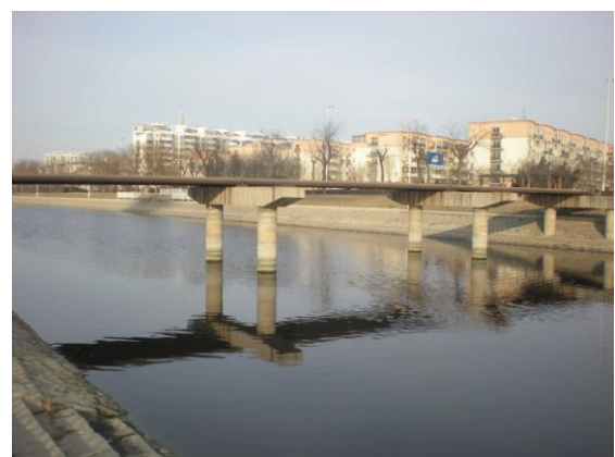
Fig. 11 Chentaizi Drainage Canal (Huayuan residential area, Xiqing District)
