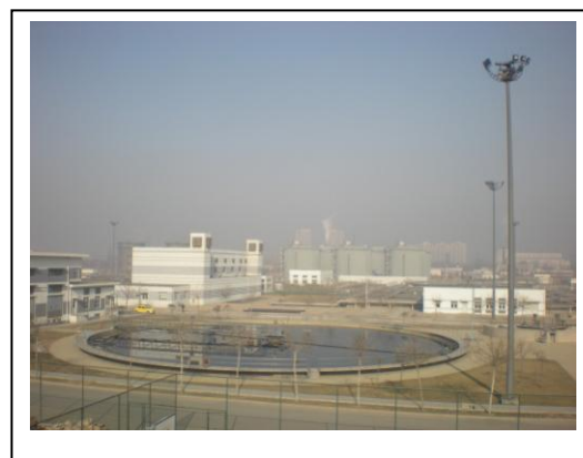
Xianyanglu Sewage Treatment Plant
