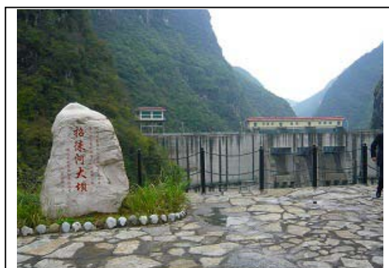
Changyang Zhailaihe Hydropower Plant
