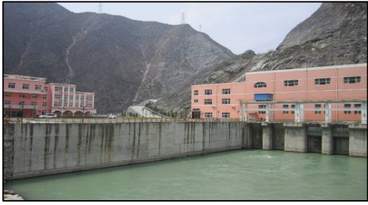
(Turbine Building, Hepingzui Hydropower Plant)
