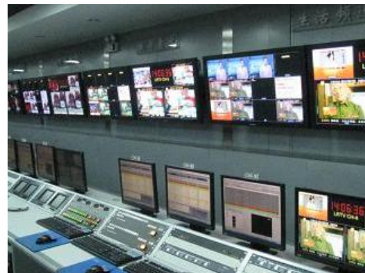
New Equipments Provided Under the Project
