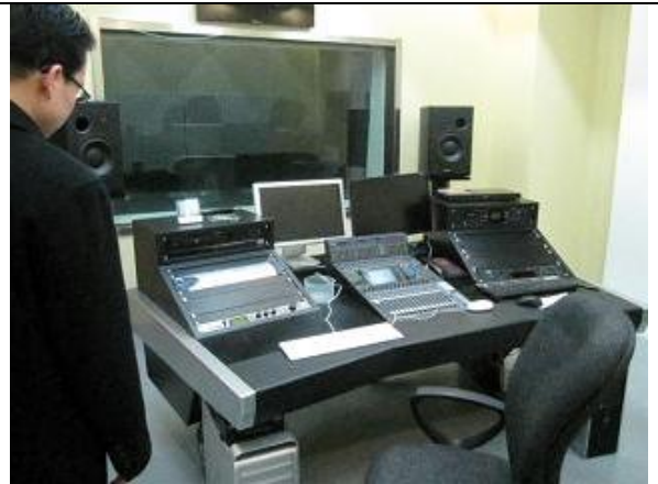
Photograph 2 Newly installed equipment (RL)
