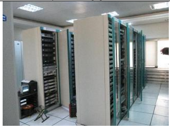
Photograph 4 Newly installed equipment (LRTTBC)
