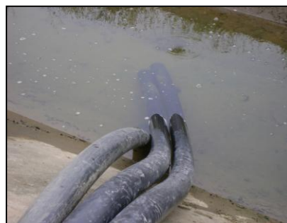
Photo 3 Direct Water Intake
