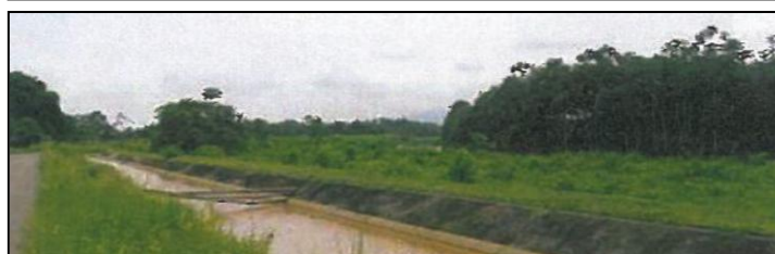
Top: Sibimbe Head Works / Bottom: Main Irrigation Channel in Sibimbe Area
