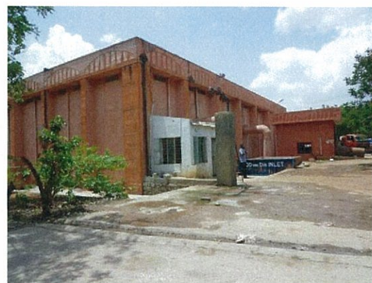
Water supply facility in Hyderabad
