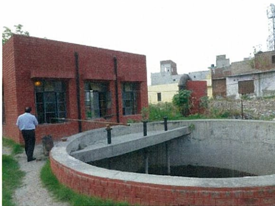
Sewerage facility in Amritsar
