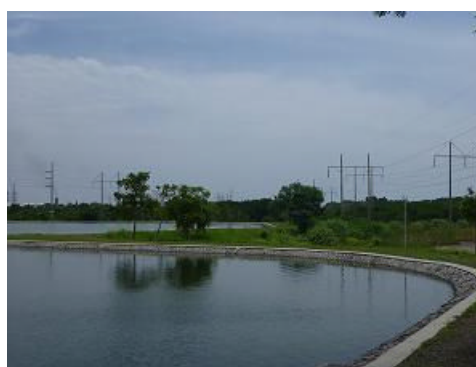
Stabilization Pond at Waste Water Treatment Plant
