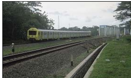
Commuter train running on the new track and steel bridge
