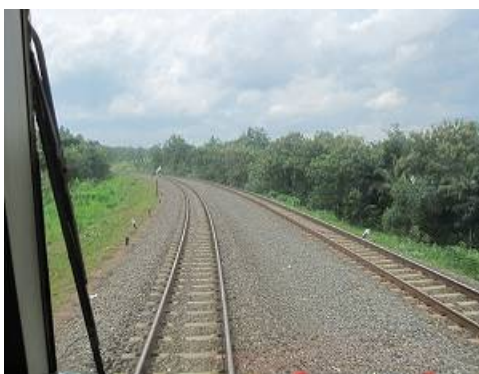
The existing track rehabilitated (right) and the new track
