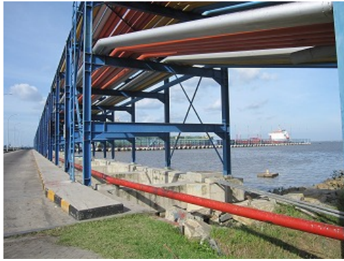
View of the palm oil wharf and pipe rack from the end of the trestle
