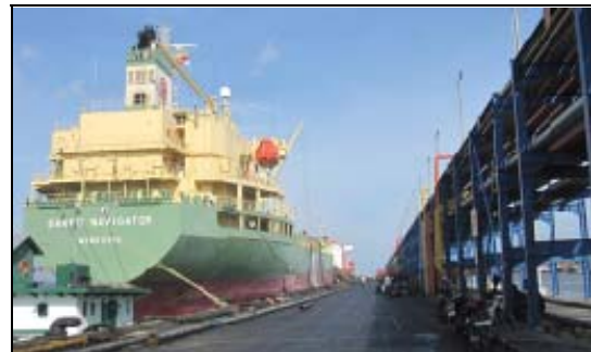
Palm oil wharf newly constructed by the project
