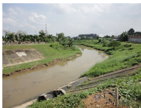
Percut River after improvement
