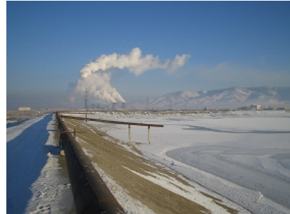
(TPP4, View from the Ash Pond)
