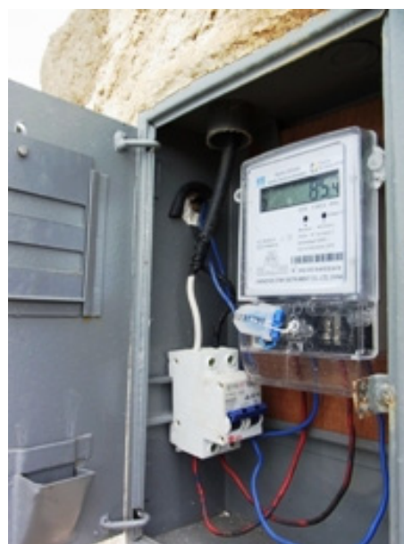
Installed Wattmeter
